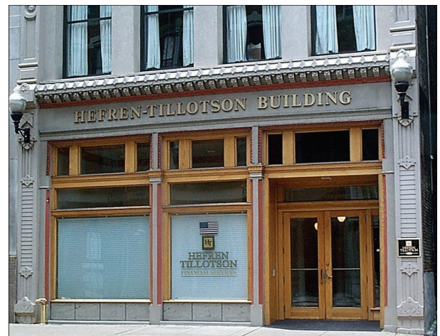
Figure 17. Storefront with commercial wood-and-glass doors
