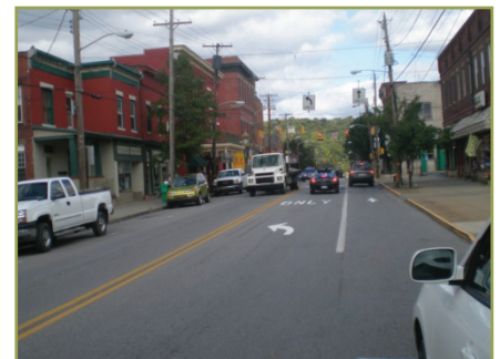
US 19 approach SR 228 - narrow lanes
