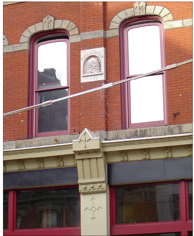
Figure 25. Stone trim cleaned and repaired
