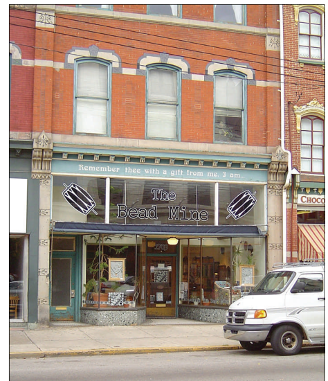
Figure 11. Storefront filled with glass
