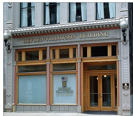
Figure 33. Signboard with individual letters and window signs
