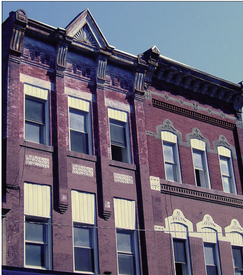
Figure 28. Inappropriately small replacement windows
