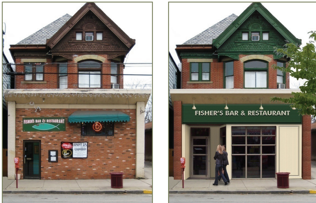
example of a façade upgrade
