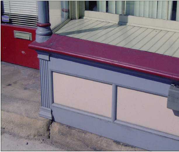
Figure 20. Paneled wood bulkhead panels below display windows
