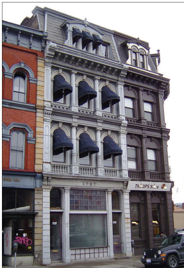
Figure 30. Awnings over window openings on upper floors
