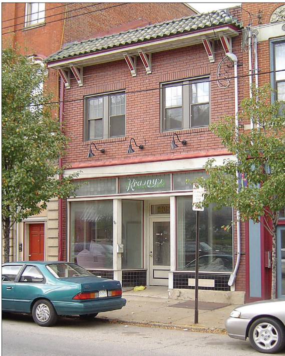
Figure 22. Tiled bulkheads below display windows
