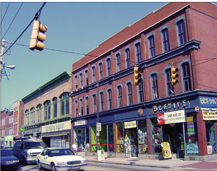
Figure 1. Intact neighborhood commercial buildings
