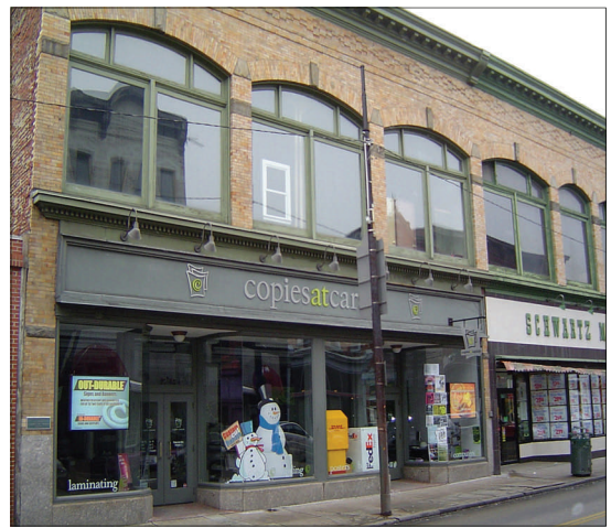
Figure 13. Storefront with signboard cornice
