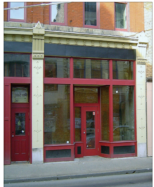
Figure 19. New storefront designed in accordance with traditional principles
