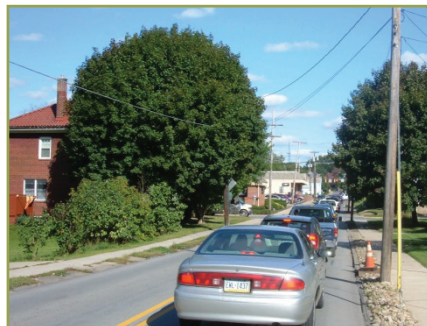
Eastbound queue on SR 68 at US
