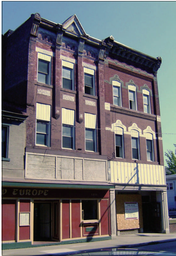
Figure 12. Storefronts with not enough glass (left) or recessed too far (right)
